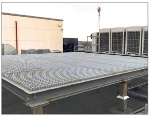
In the long run. The high strength-to-weight ratio of fiberglass grating surprises those in charge because it is both light and strong. It provides a light but strong surface that helps protect the structural integrity of the roof. Elevated flooring systems allow rainwater and other liquids to drain efficiently through the synthetic turf into the roof surface. In addition, the raised floor system can be extended to a fenced off dog park for pedestrians to enjoy.
